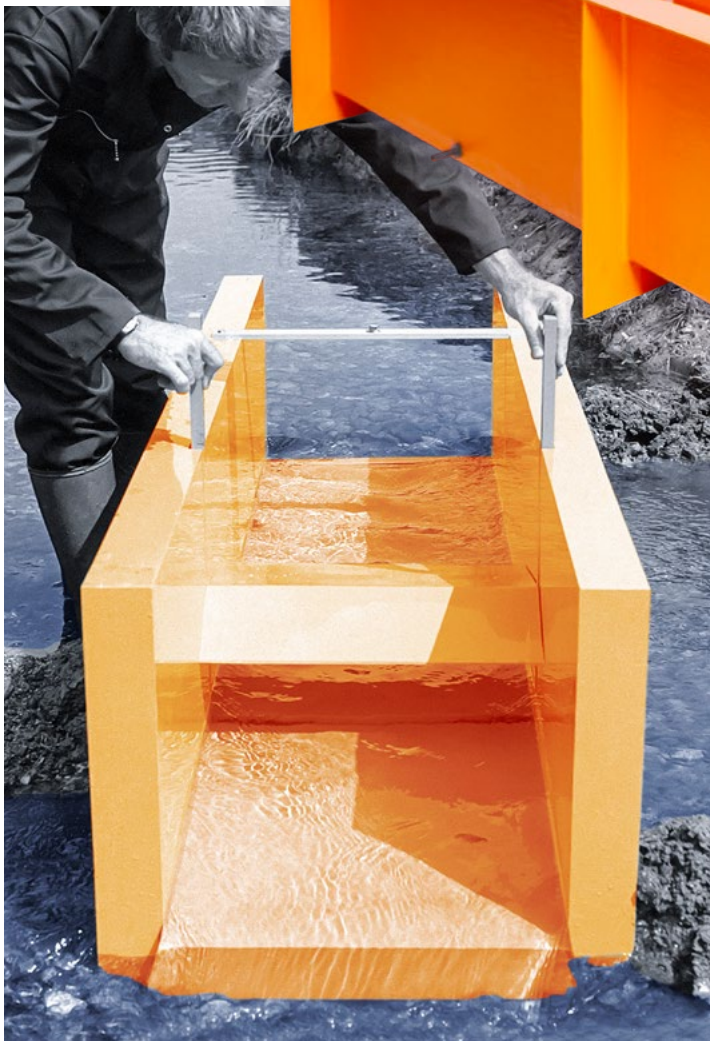
FEX26-11 Crump Weir being fitted, see page 3
